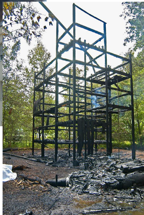
Fig. 8: Burnt-out climbing frame in the adjacent playground
